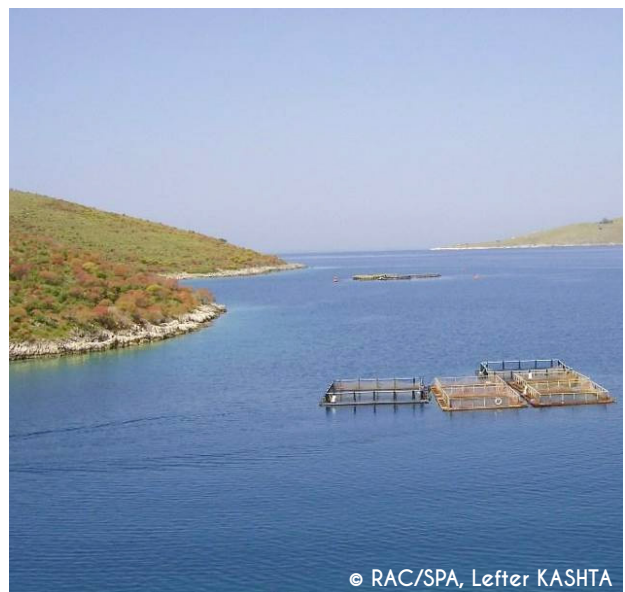
Figure 28. Fish farm infrastructures within the Porto Palermo bay
